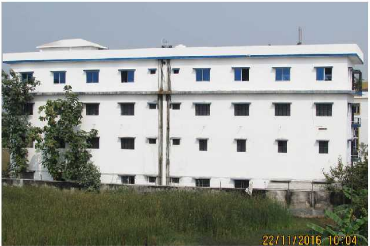
Rear view of the building
